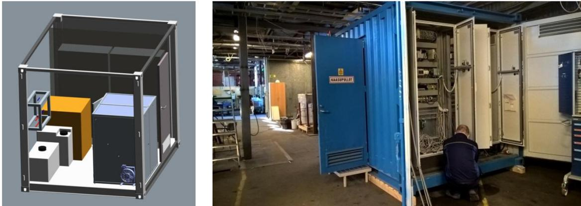
Figure 6: REFCS container layout (left) and photo with the automation system installation in progress (right).
